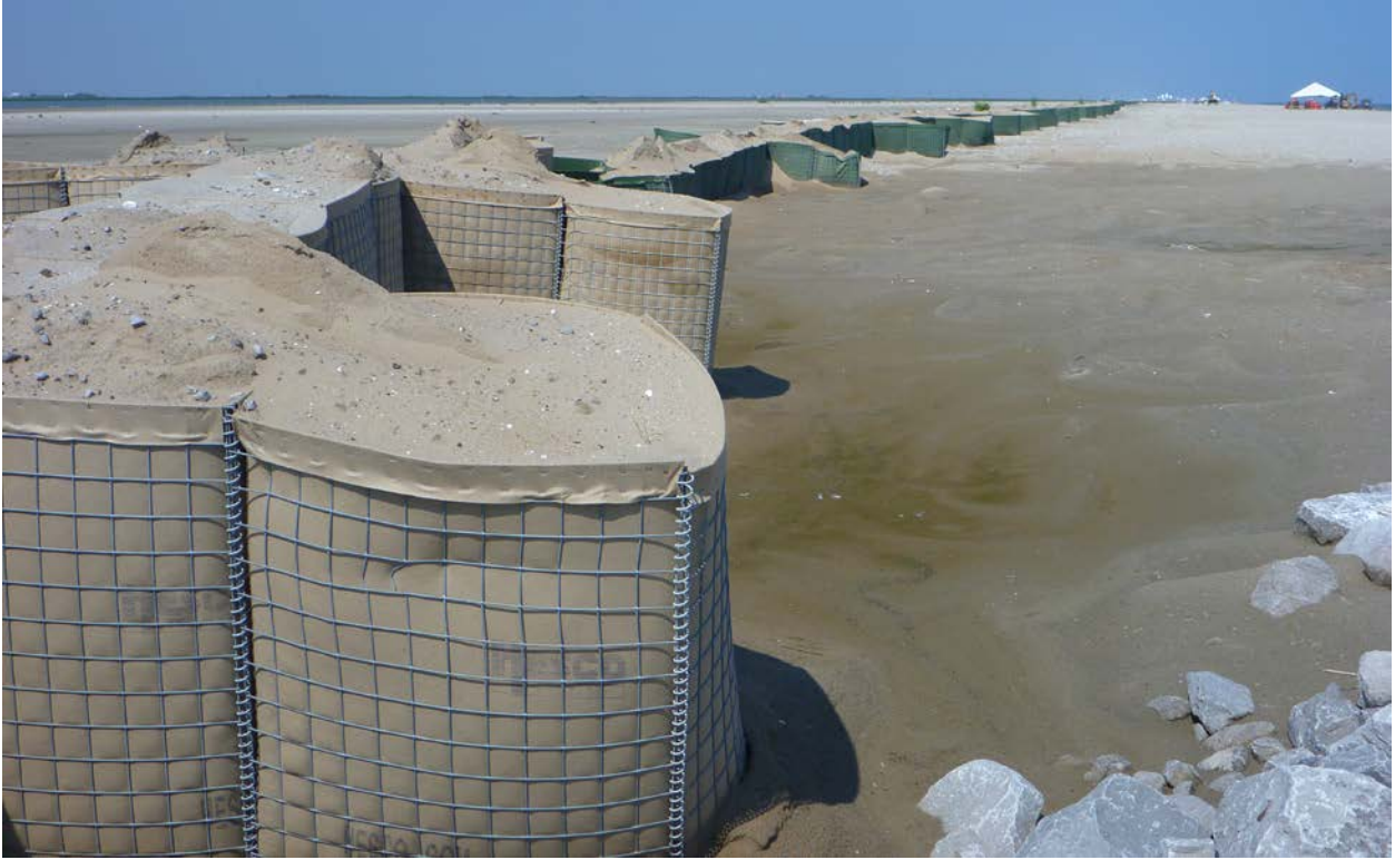
Figure 4.3C Close up view of armored baskets filled with sand.
