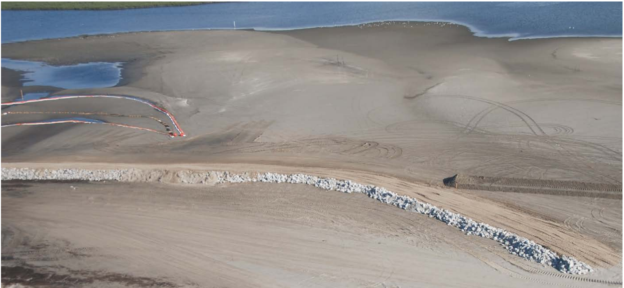
Figure 4.4 Rip-rap revetment protecting a tidal flat and back bay.
